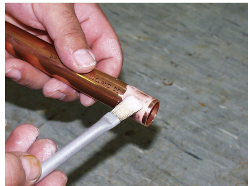
4. Apply the soldering flux on the pipe
